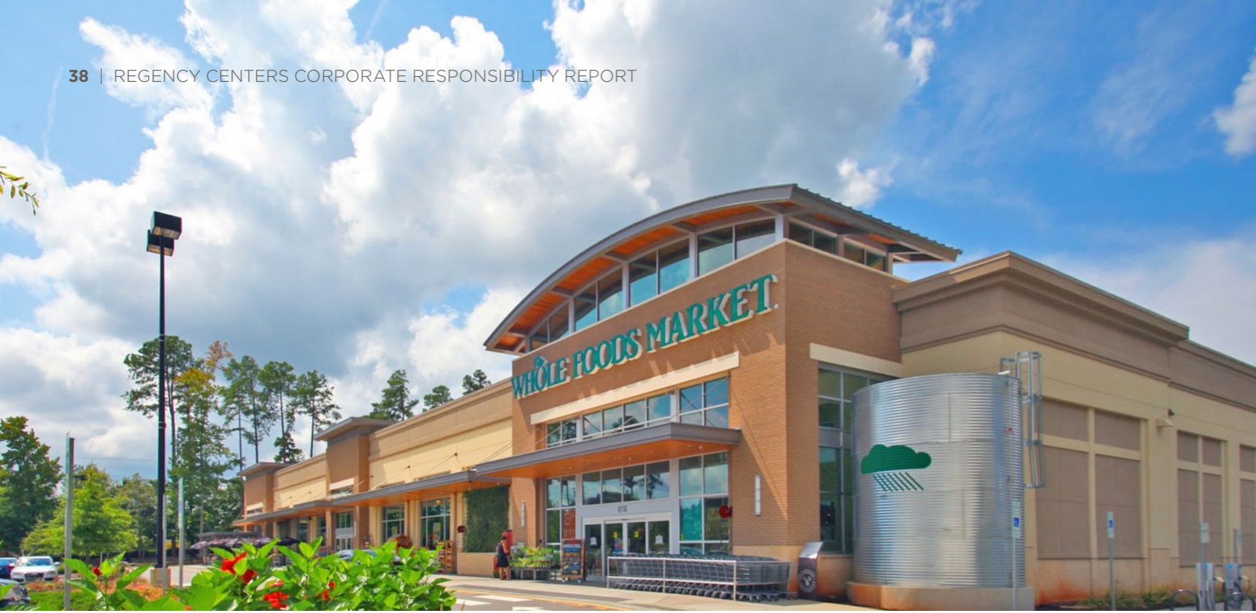
Market at Colonnade Center | Raleigh, NC | Above-Ground Cistern
