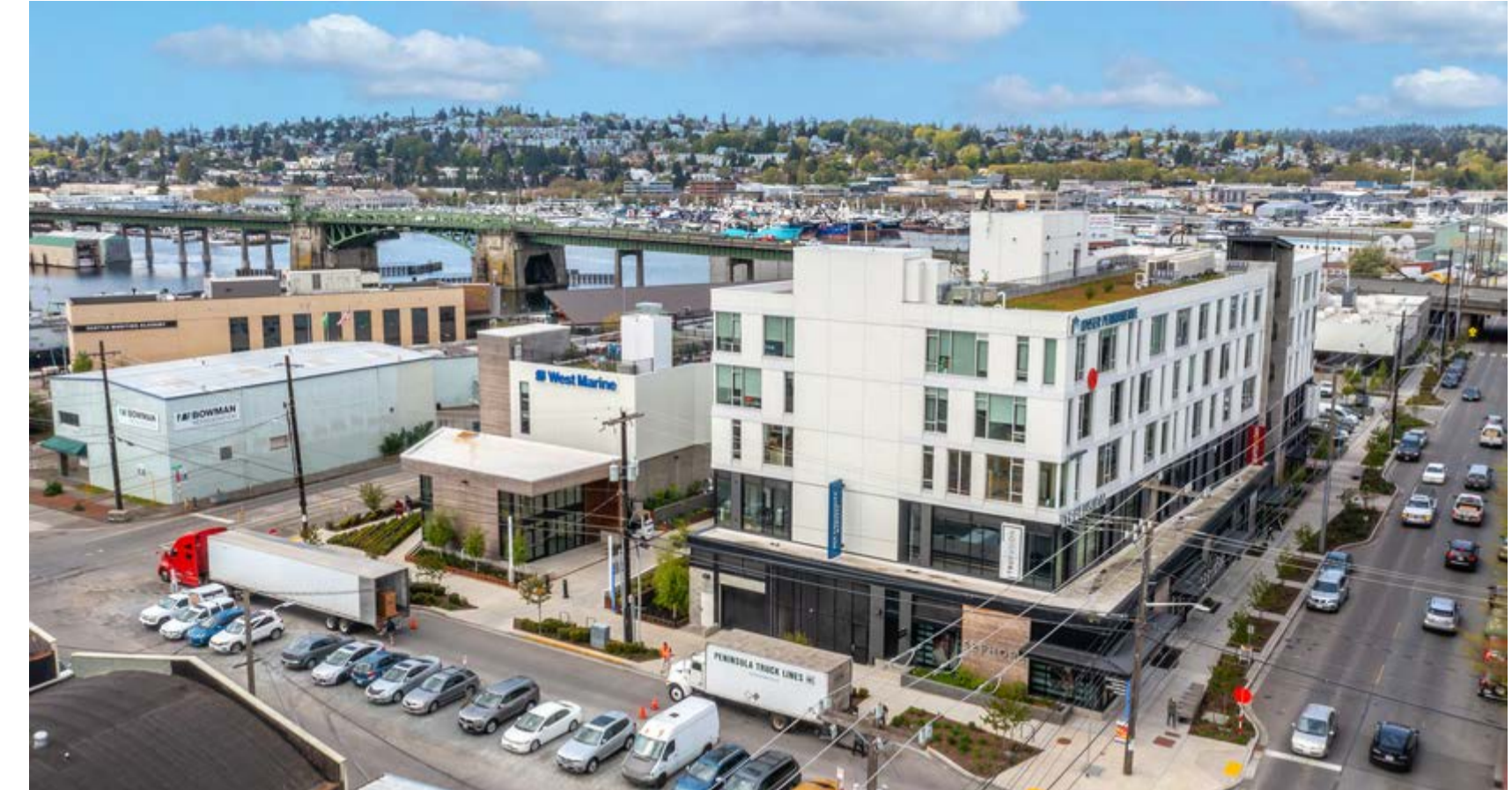
Ballard Blocks I | Seattle, WA | LEED Silver
