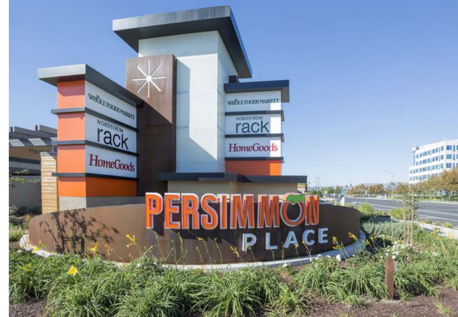
Persimmon Place | Dublin, CA LEED Gold
