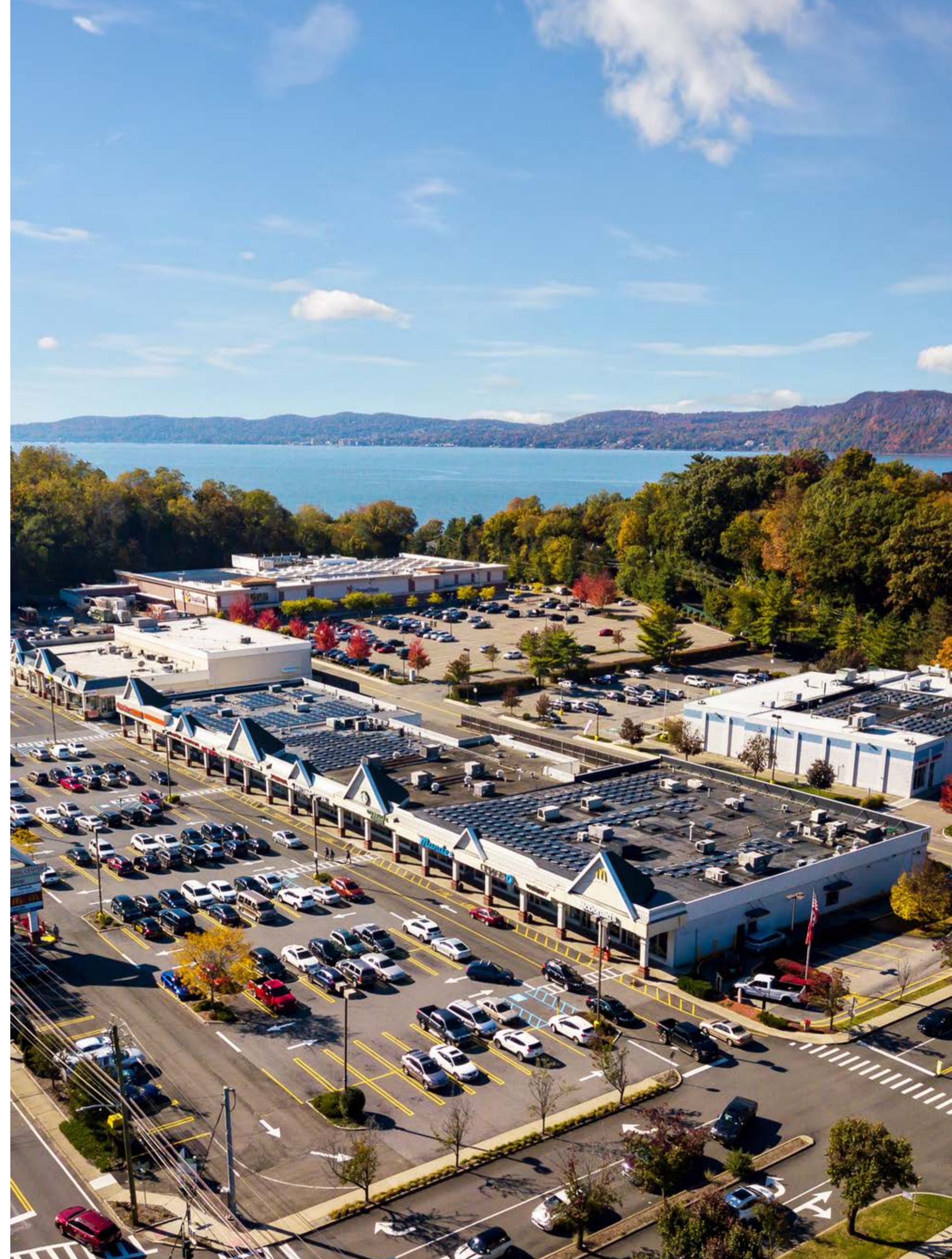
Arcadian Shopping Center | Ossining, NY
