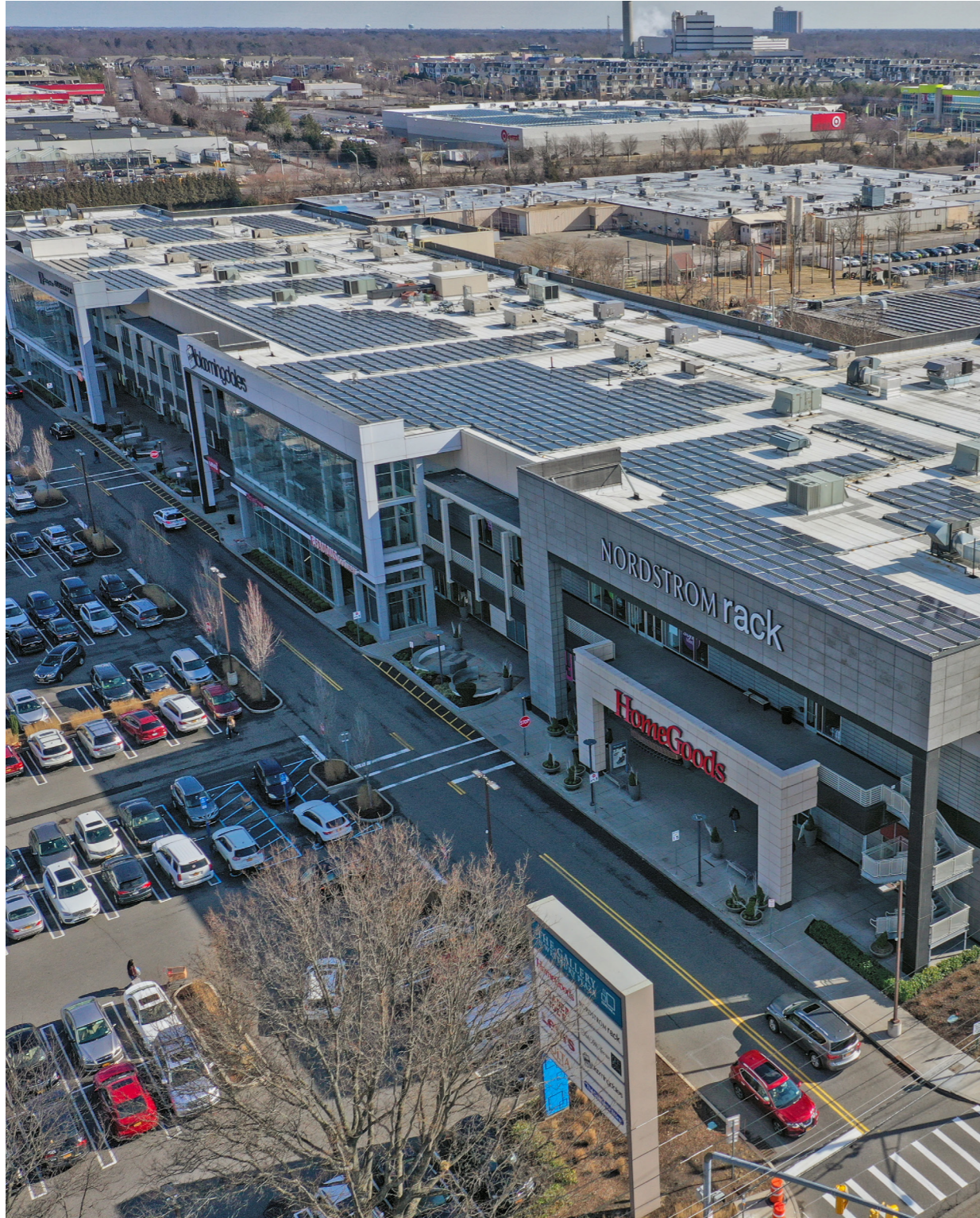
The Gallery At Westbury Plaza | New York, NY | Rooftop Solar Panels
