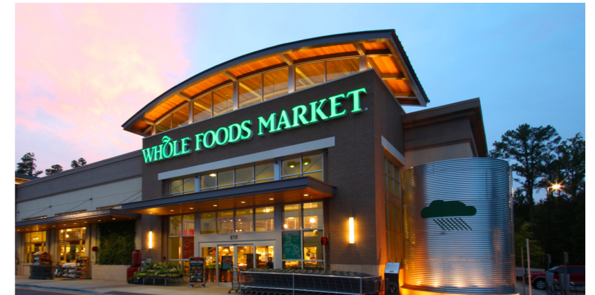
Market at Colonnade Center | Raleigh, NC | Rainwater Cistern
